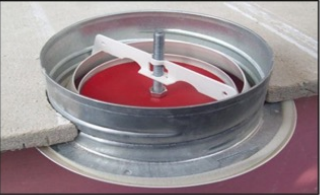
Fire Rated Ceiling Valve installed before a fire.
