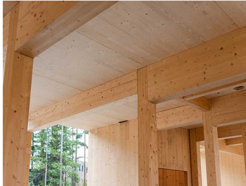
Panelised 2D - Post & Beam CLT
