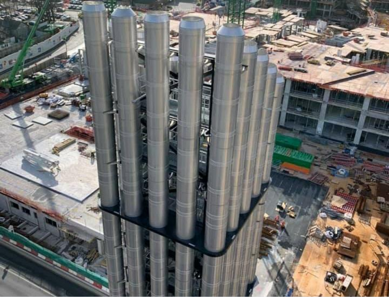
BAM Ireland – National Children's Hospital Modular Flue stack
