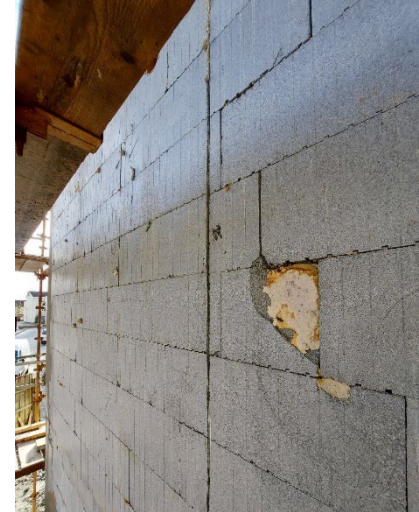
(2) WALLS: EXTERNAL INSULATION ON SOLID MASONRY/HOLLOW BLOCK
