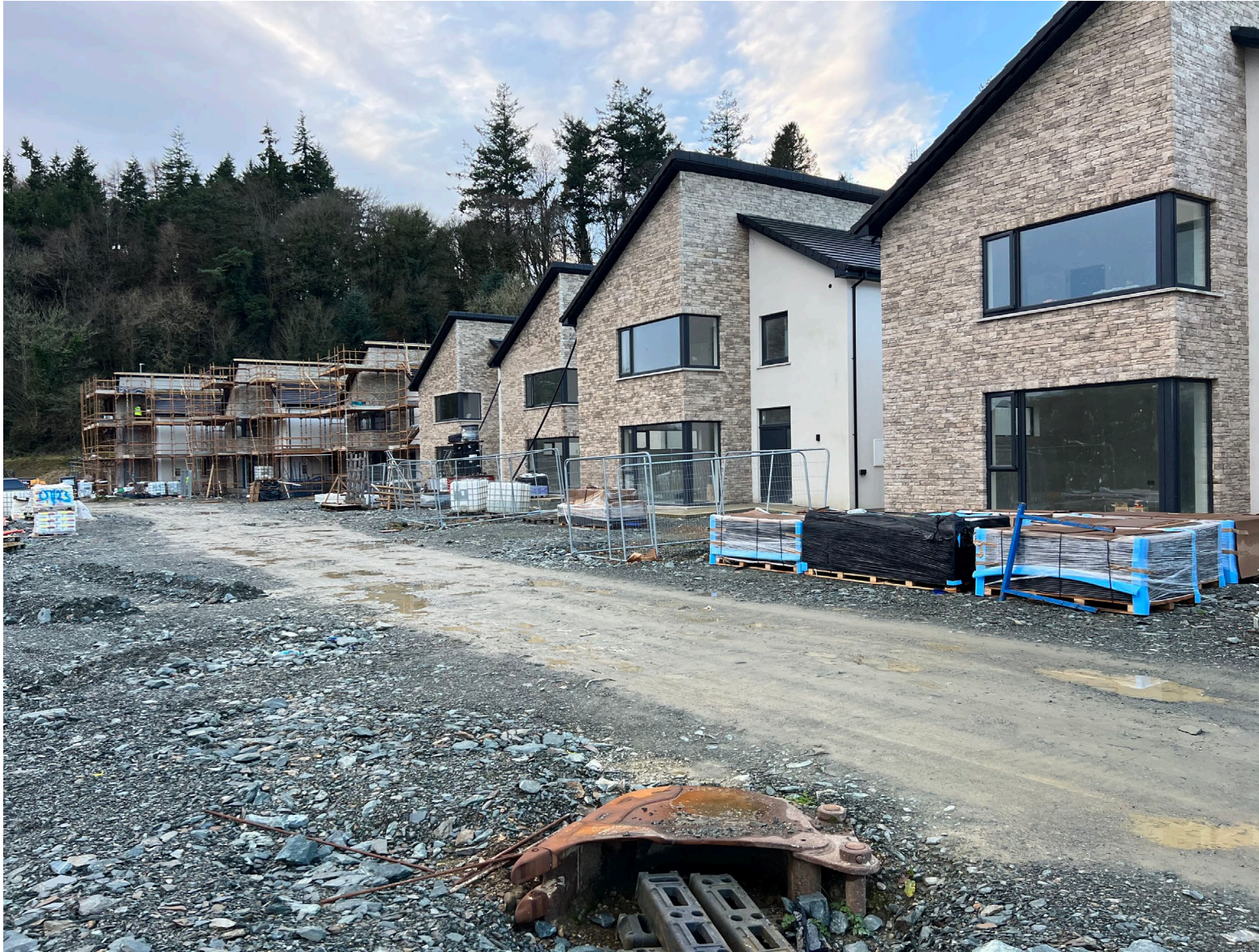
Recent build with raft foundations + ICF – Rathdrum
