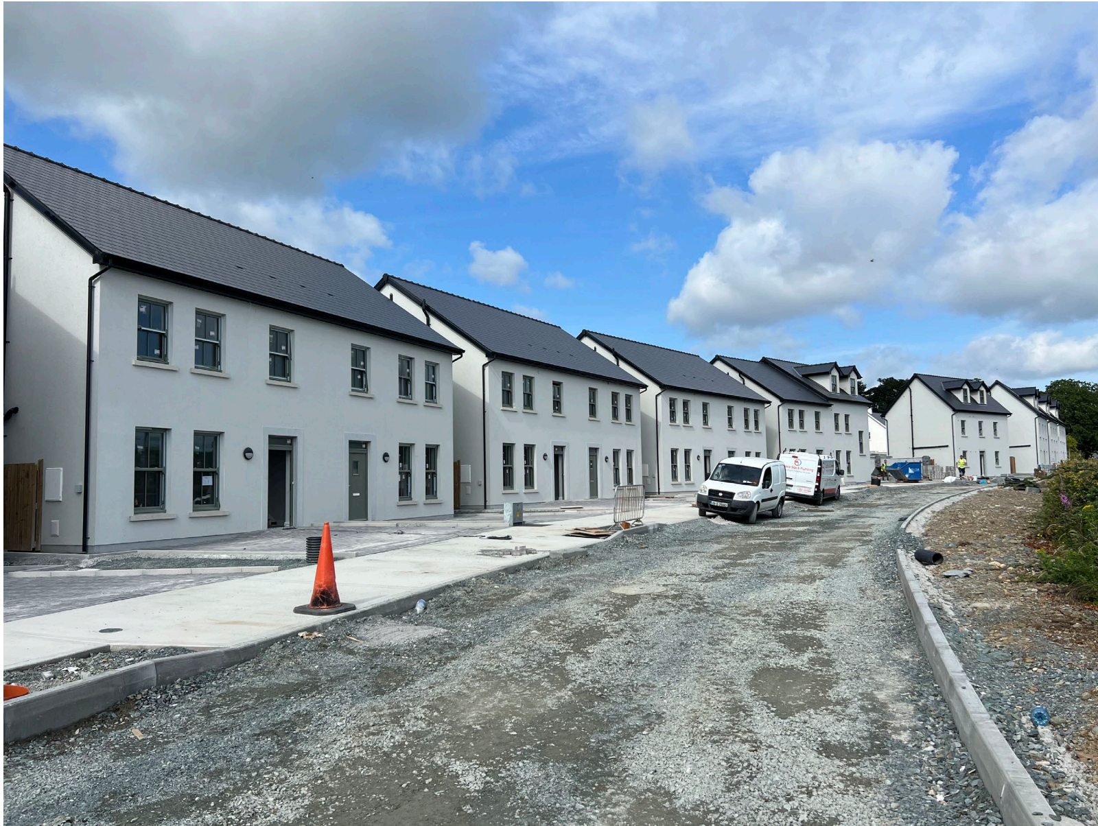
Recent build with raft foundations + timber frame – Newcastle
