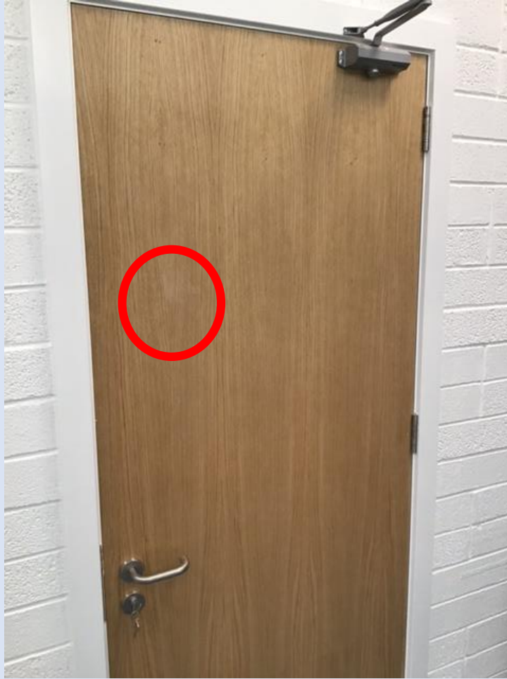
Fire door plaque missing
