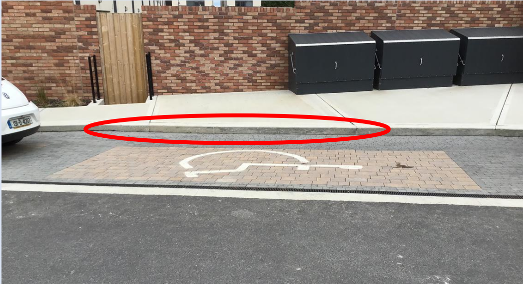
No dropped kerbs
